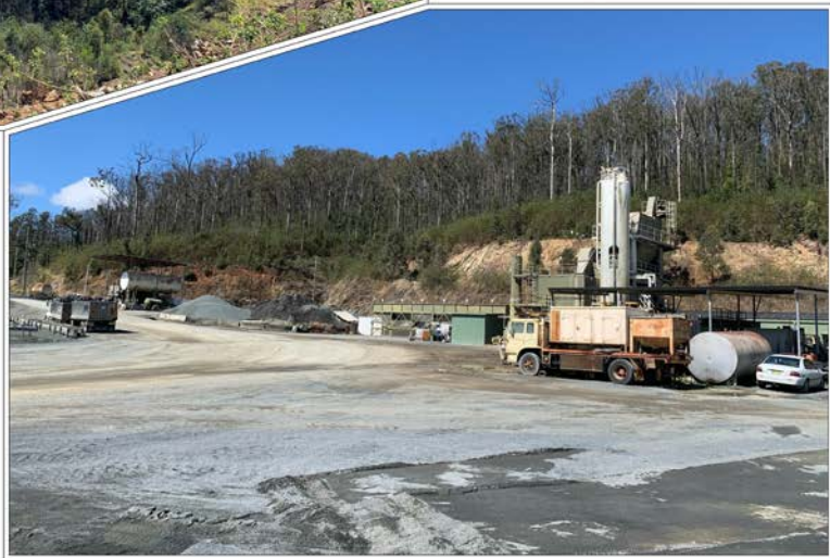
Plate 10: View to the southeast towards the Asphalt Plant
