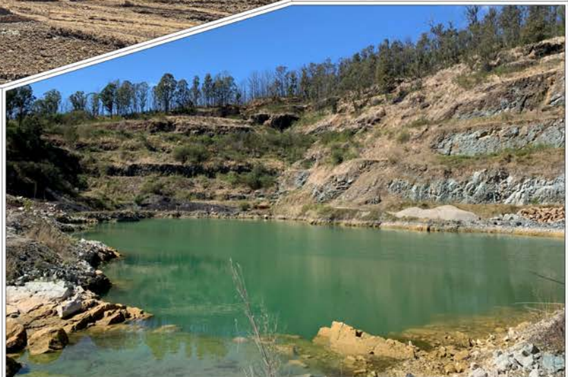
Plate 4: View to the southeast of the Area A sump and rehabilitated benches in the background.
